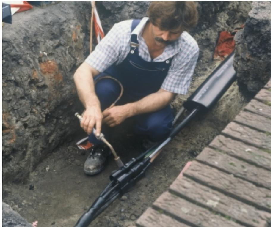
The conductors can be jointed with either mechanical, compression or soldered connectors, which are then insulated by shrinking adhesive-lined thick-walled tubing over them, at the same time finally sealing the cores of both cables.
