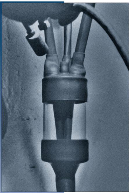
The tough transparent oil reservoir allows easy inspection and maintenance and is fitted with outlets of heat-shrinkable material, internally pre-coated with adhesive. In this photo the lower end has already been shrunk onto the lead cable sheath, and the upper outlets are seen being shrunk onto the cable cores, which have been protected from humidity and dust with rigid heat-shrinkable tubing.
