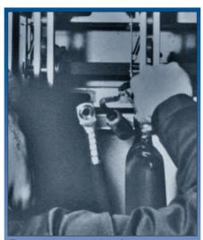
To seal the transition from connecting lug to cable core, sealing sleeves pre-coated with adhesive are shrunk into place. The termination need only be filled with oil and connected before power can be energized.
